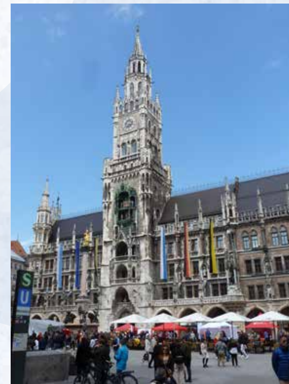
The Neues Rathaus (New Town Hall) Munich
